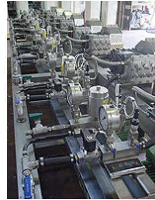
View of a typical pump rack (number of pumps up to five).
