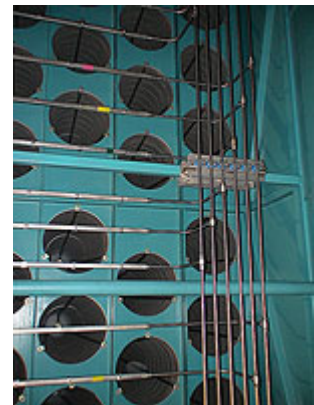
Portion of the inside nozzle rack (in the background are the air filters).
