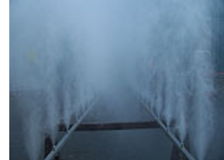
Example of water injection from EnergyFog nozzles.
