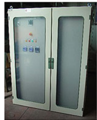
I&C cabinet, which includes the pump inverters.
